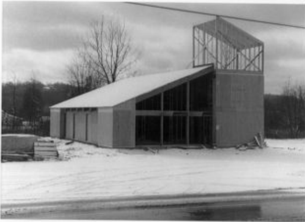
New church under construction – January – March 1969
